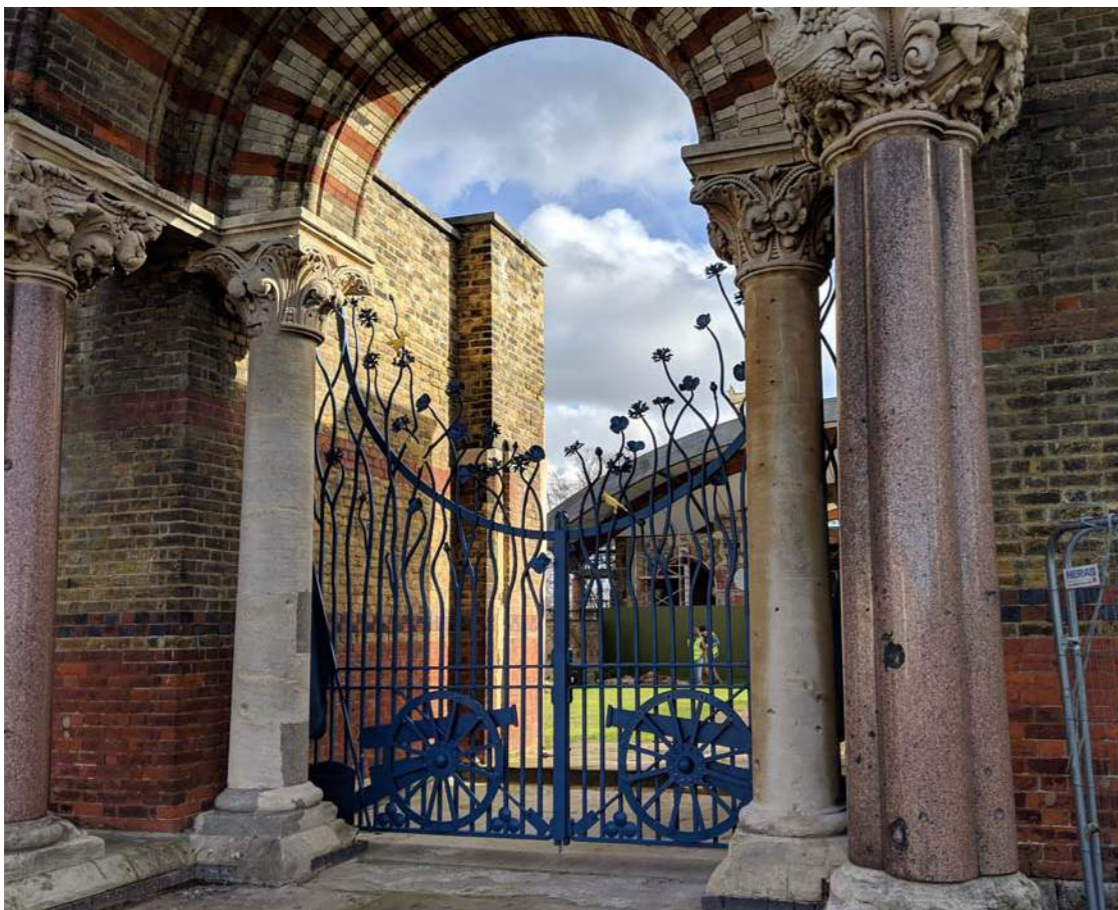
Below: Front Entrance with new gates, opened by HRH The Duke of Gloucester.
