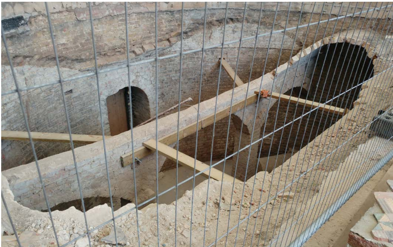
Below: Phase 2 Excavating the Crypt, which had filled with debris from the bombed church tower above.
