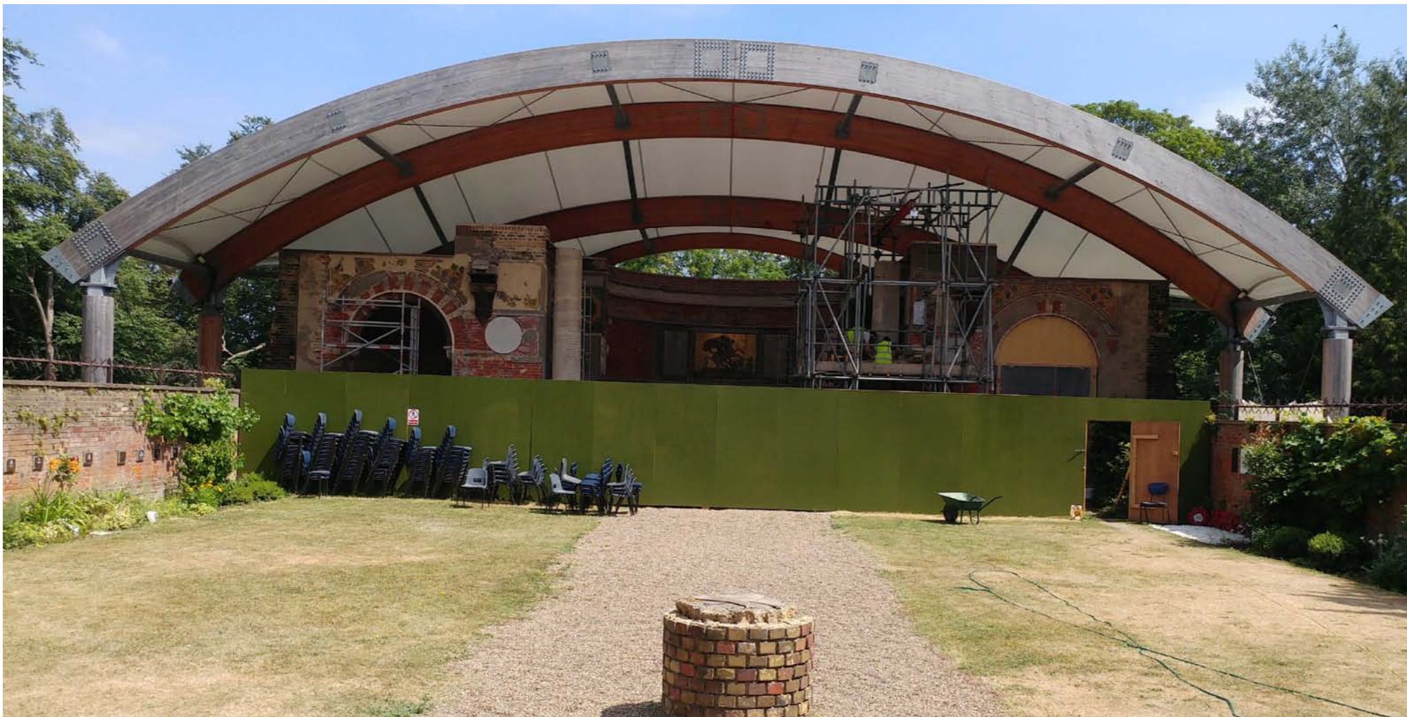
Above: Phase 1 canopy and the Phase 2 restoration works ongoing below.
